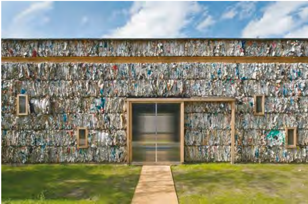
Figure 2: Dratz & Dratz Architects, PHZ2 Project , 2008-2010, Essen, Germany, recycled paper, wood (Basural n.d.).
