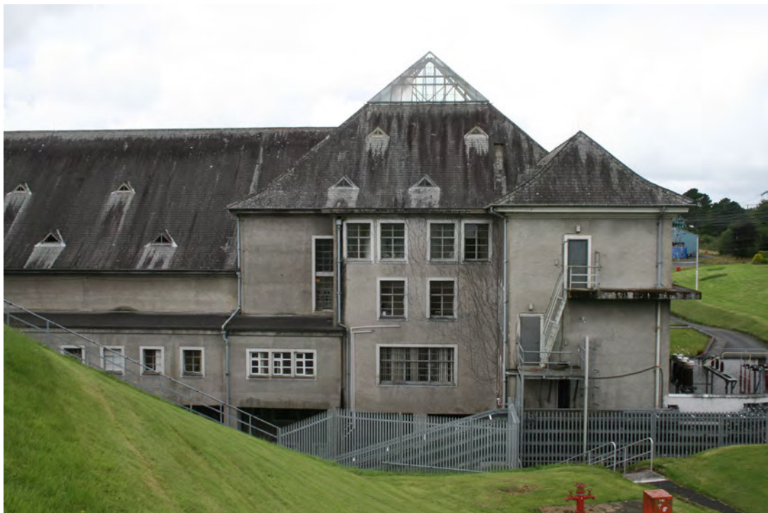
FIGURE 3-18 - REAR OF ARDNACRUSHA ADMINISTRATION BUILDING, WITH TURBINE HALL AND 10KV SWITCH HOUSE EXTENDING TO THE LEFT (PHOTOGRAPH TAKEN BY THE AUTHOR, AUGUST 2008)
