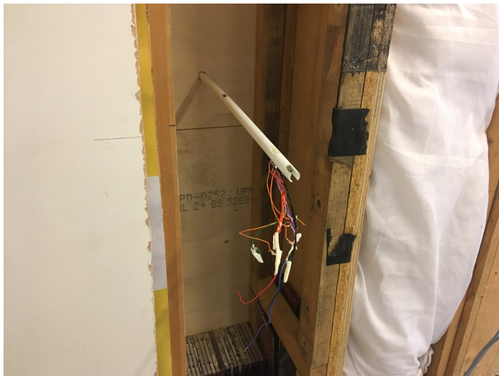
(a) Probe installation
