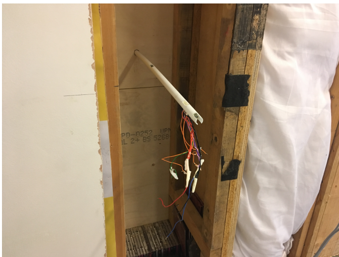
(a) Probe installation
