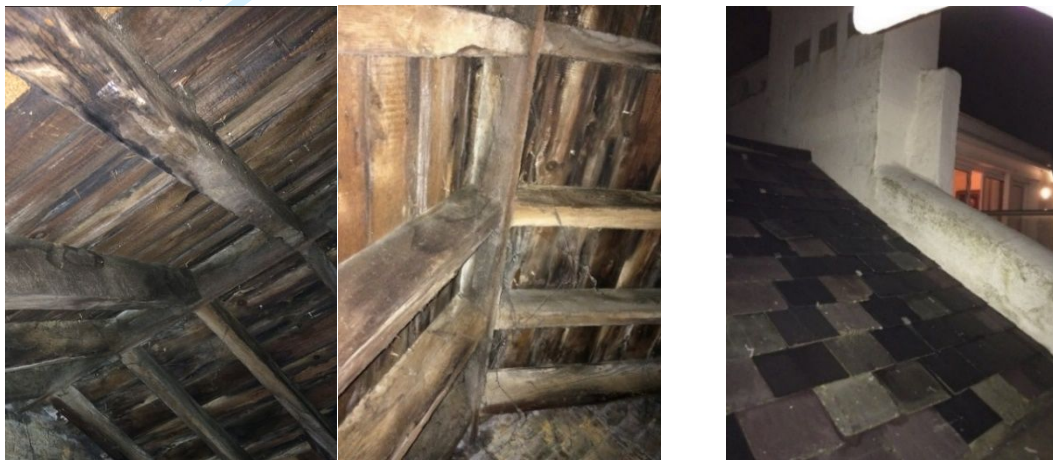
FIGURE 0.2 THE TIMBER ROOF IN CS7 -INSIDE AND OUTSIDE- SHOWING THE TIMBER CONSTRUCTION AND THE SLATE TILES CLADDING
