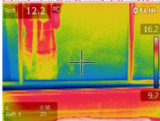
5 THERMOGRAM 3: THE SASH WINDOW IN THE GUEST BEDROOM, SHOWING THE AIR LEAKAGE TAKING PLACE THROUGH THE WINDOW FRAME.
