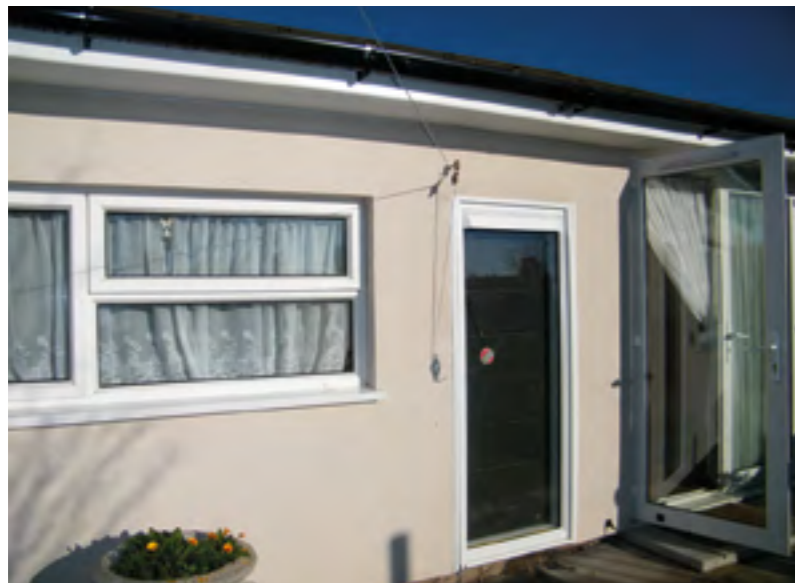
The Rushenden Trombe wall fits into traditional building design.
