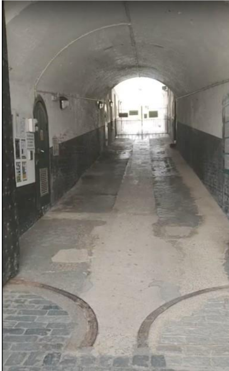
Fig. 7.23: Newhaven Fort entrance tunnel, November 2019. Image: Harriet Parry.
