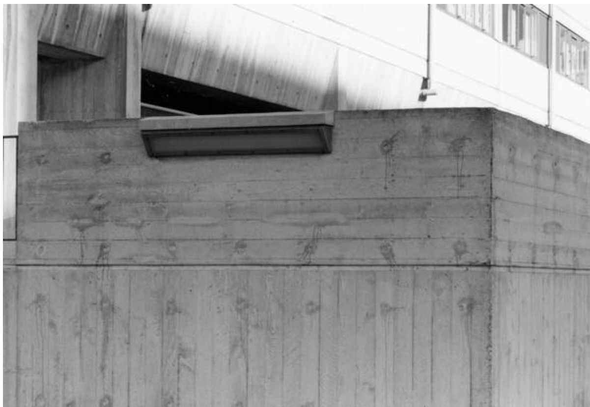
Fig. 3.20: Detail of 'sawn finish' style concrete. Taken from 'Ramp along south elevation'. Photo by Rose and Dyble, circa 1969. Image: RIBA Archive.
