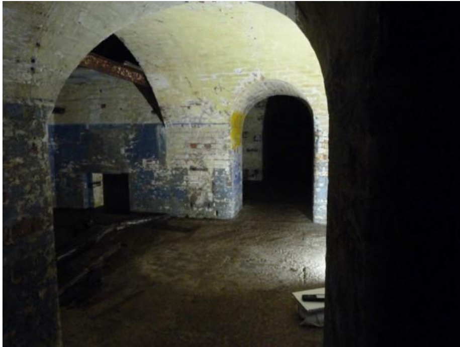
Fig. 7.20: Northwest counterscarp galleries (now closed for safety), March 2018. Image: Harriet Parry.
