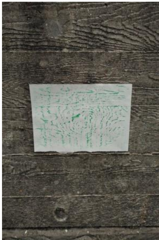
Fig. 5.5: Wyndham Court 'sawn-timber' concrete texture rubbing, May 2019, Harriet Parry.
