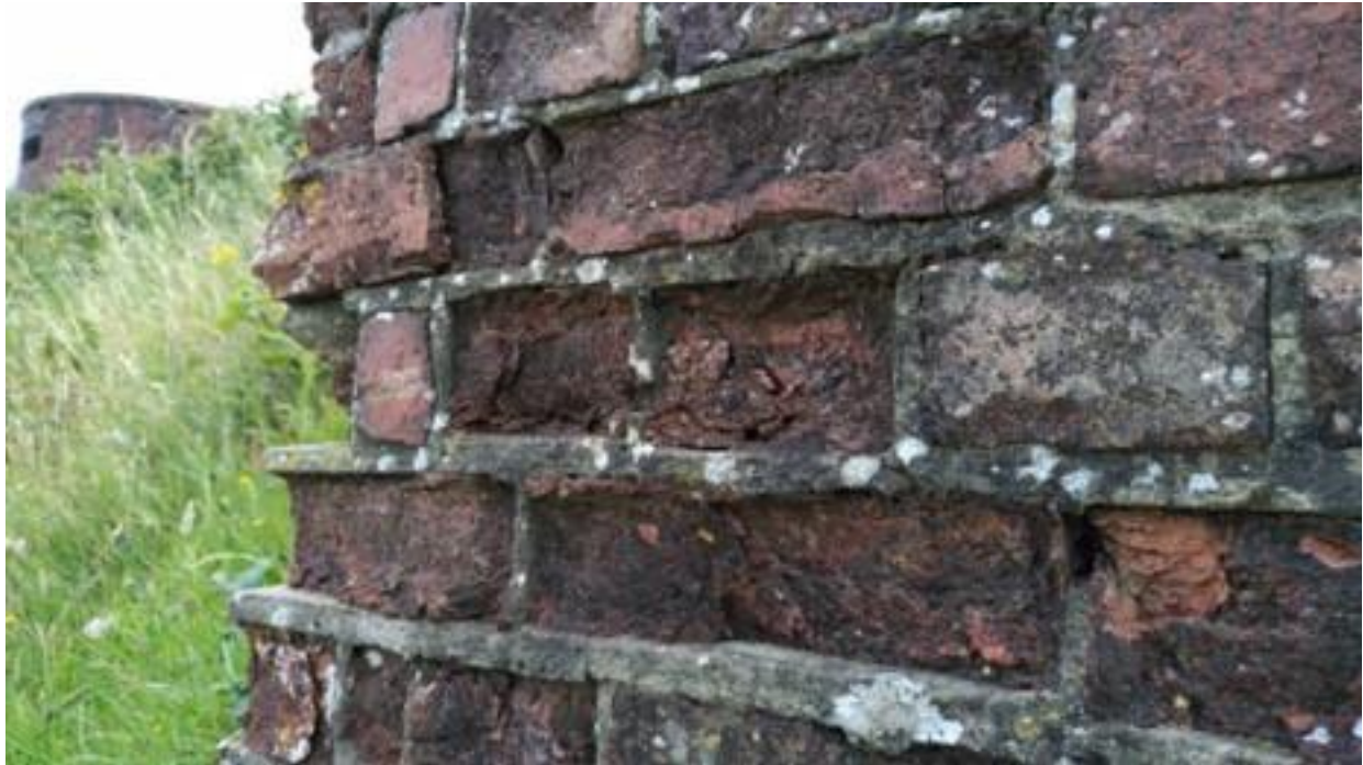
Fig. 7.22: Brick and grass at Newhaven Fort, 2021. Image: Harriet Parry.
