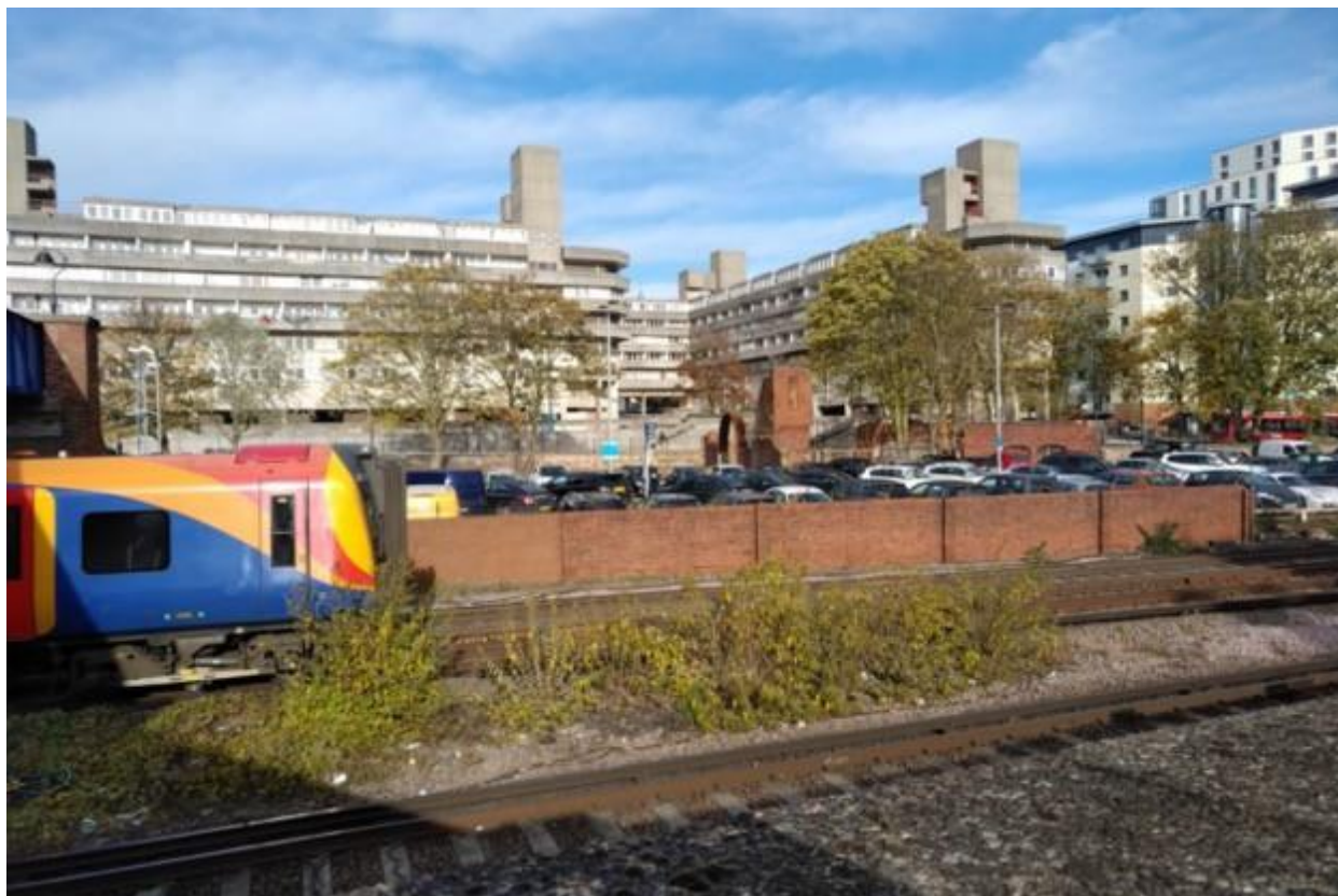
Fig. 6.3: Wyndham Court from the south side of Southampton Central station, November 2018. Image: Harriet Parry.
