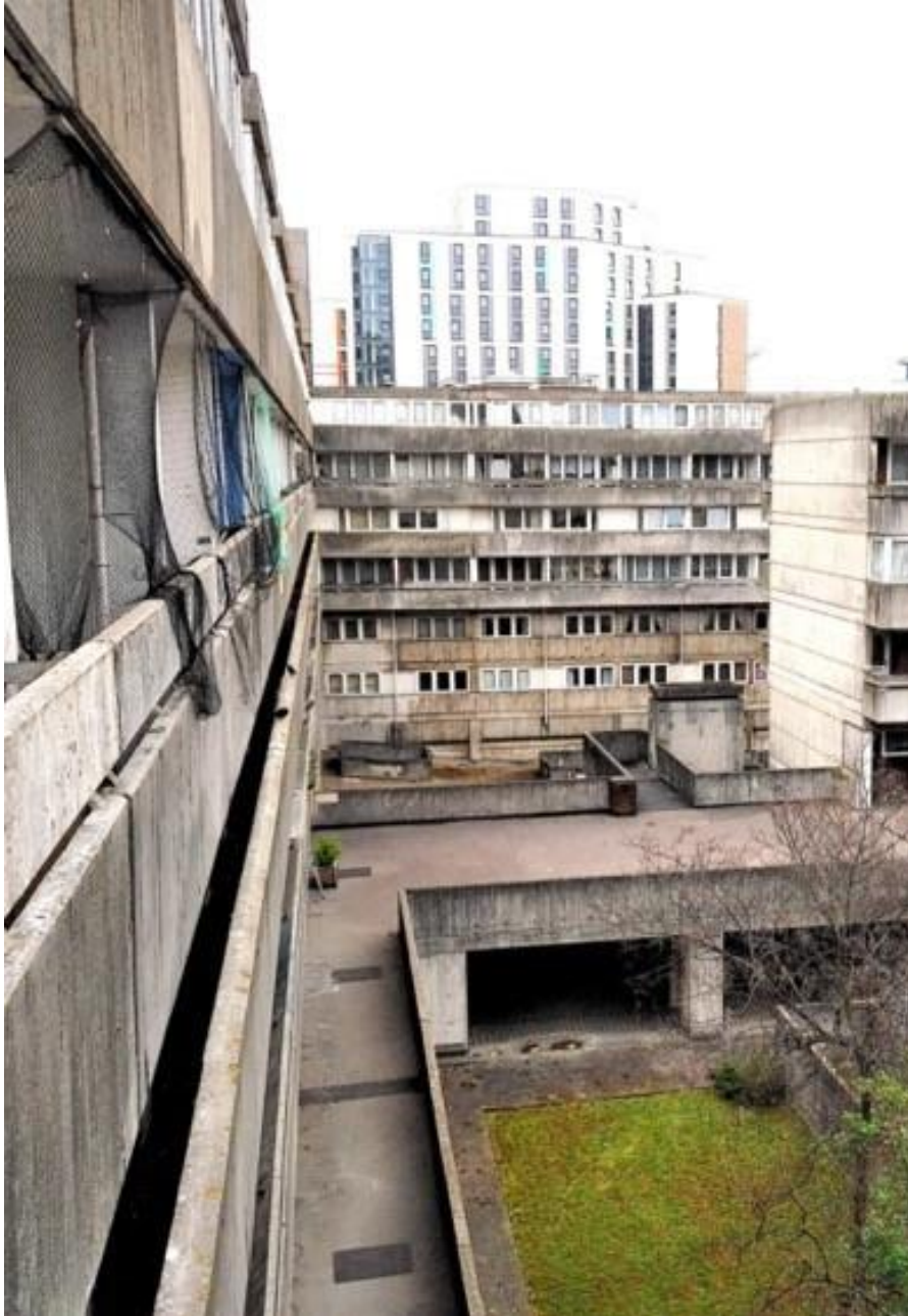
Fig. 6.28: Netting across the front of people's balconies to deter pigeons, facing Wyndham Court's interior Garden Court, September 2019. Image: Harriet Parry.
