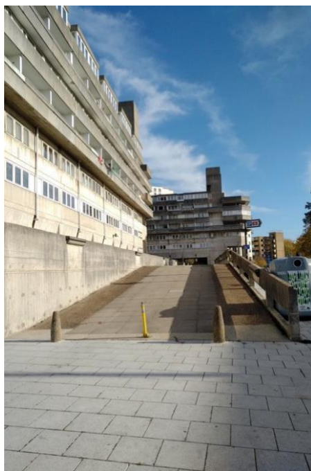
Fig. 6.6: Wyndham Court's pedestrian ramp looking east, November 2018. Image: Harriet Parry.
