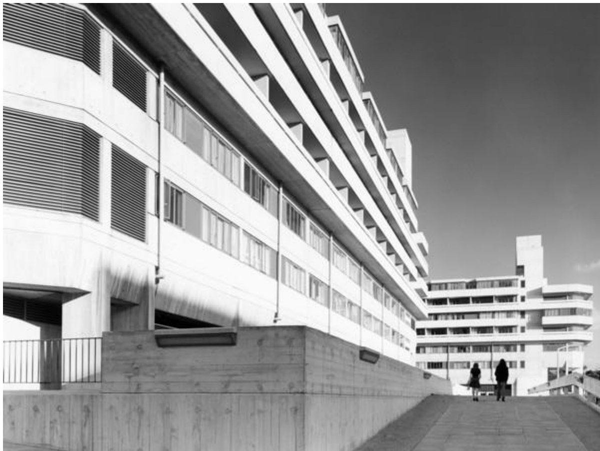
Fig. 3.19: 'Ramp along south elevation' architectural completion image. Photo by Rose and Dyble, circa 1969. Image: RIBA Archive.
