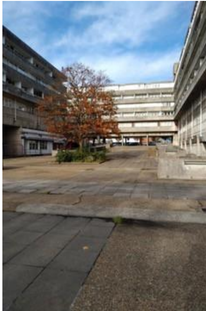
Fig. 6.34: Wyndham Court's public court, November 2019. Image: Harriet Parry.
