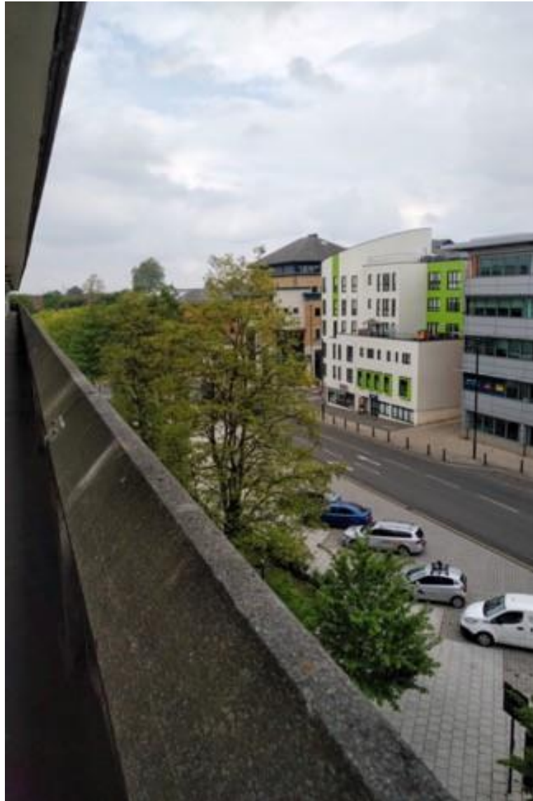
Fig. 2.14: View from the third floor pedestrian walkway of Wyndham Court looking west, September 2019. Image: Harriet Parry.
