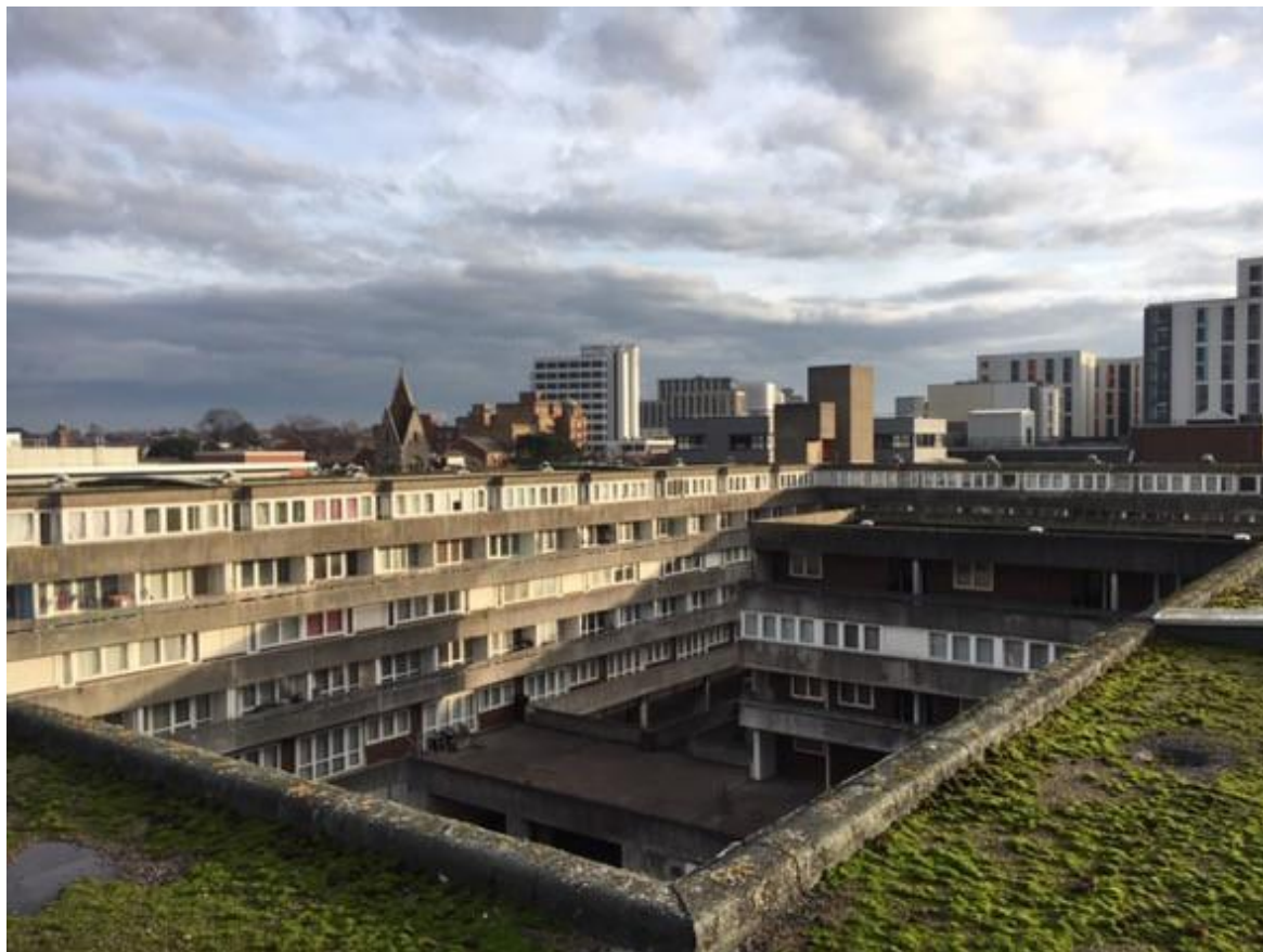
Fig. 2.16: View from the roof of Wyndham Court looking northeast, November 2019. Image: with Luke's kind permission.
