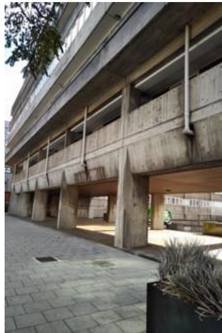
Fig. 6.36: Raised pilotis from north side on Commercial Road, November 2019. Image: Harriet Parry.
