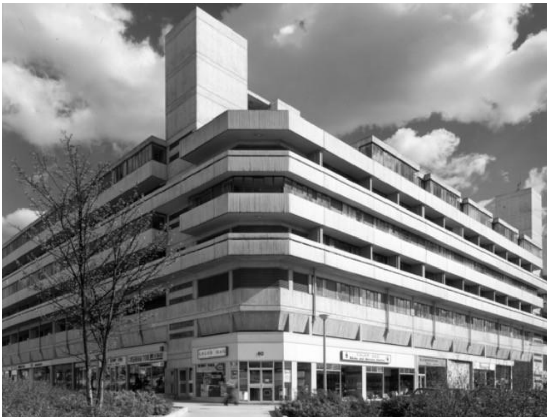
Fig. 6.37: Wyndham Court completion image of the northwest corner on Commercial Road, showing the arcade of shops. Photo by Rose and Dyble, circa 1969. Image: RIBA Archive.
