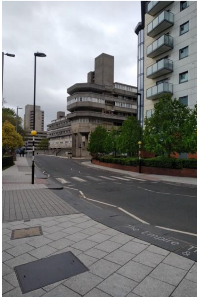
Fig. 6.41: Wyndham Court from the southeast looking west along Blechynden Terrace, April 2019. Image: Harriet Parry. Also see Rose and Dyble's completion image, fig. 6.26.
